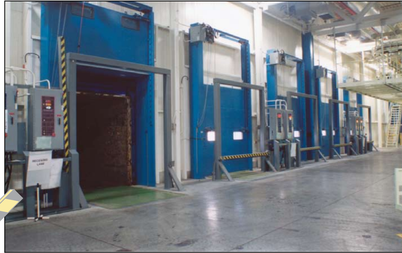
Kelley Safety Gates can be interlocked with truck restraints and are designed to operate after the truck is locked firmly in place.
